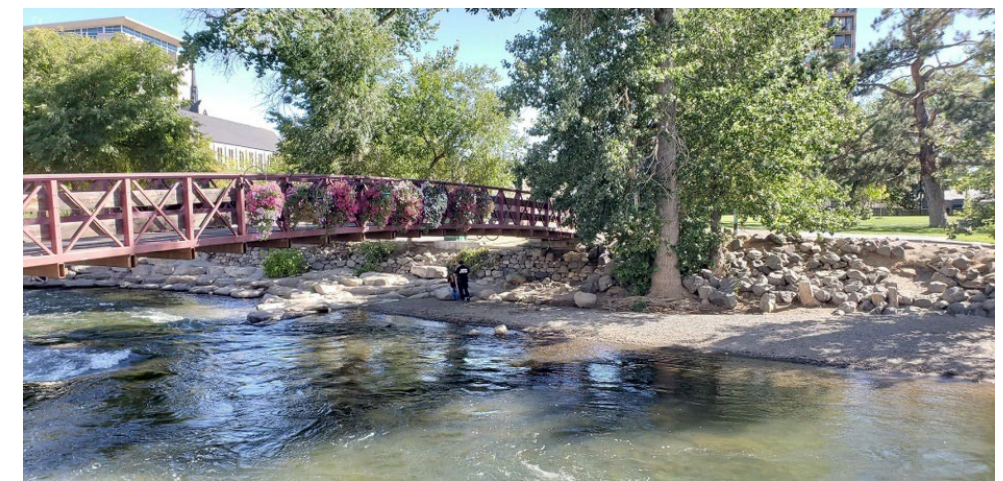
6. Pedestrian Bridge over North Branch Truckee River
