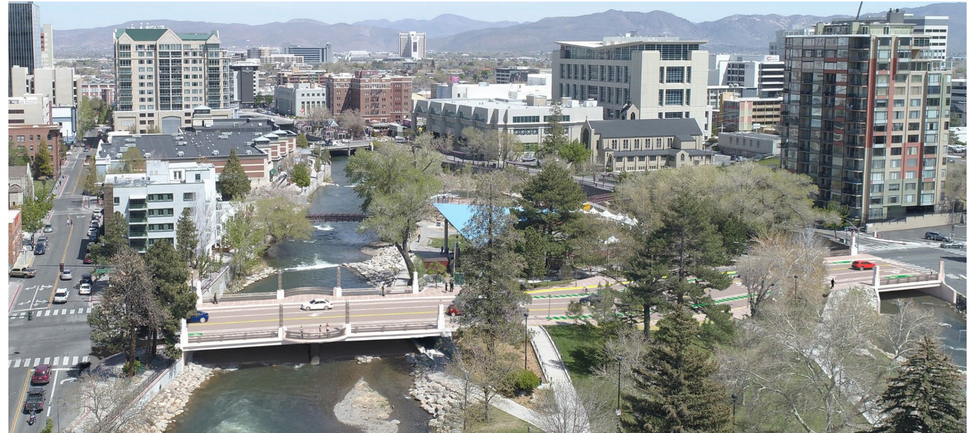
Arlington Avenue Bridges Replacements – Aerial View Looking East at both north and south branches of the Truckee River with Wingfield Park between. Source: Jacobs and Stantec Consulting, 2024
