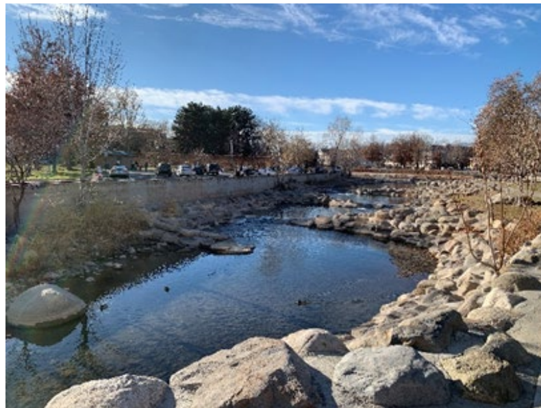
3. Floodwall and South Branch Truckee River
